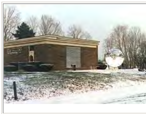
New Haven, CT Installation
